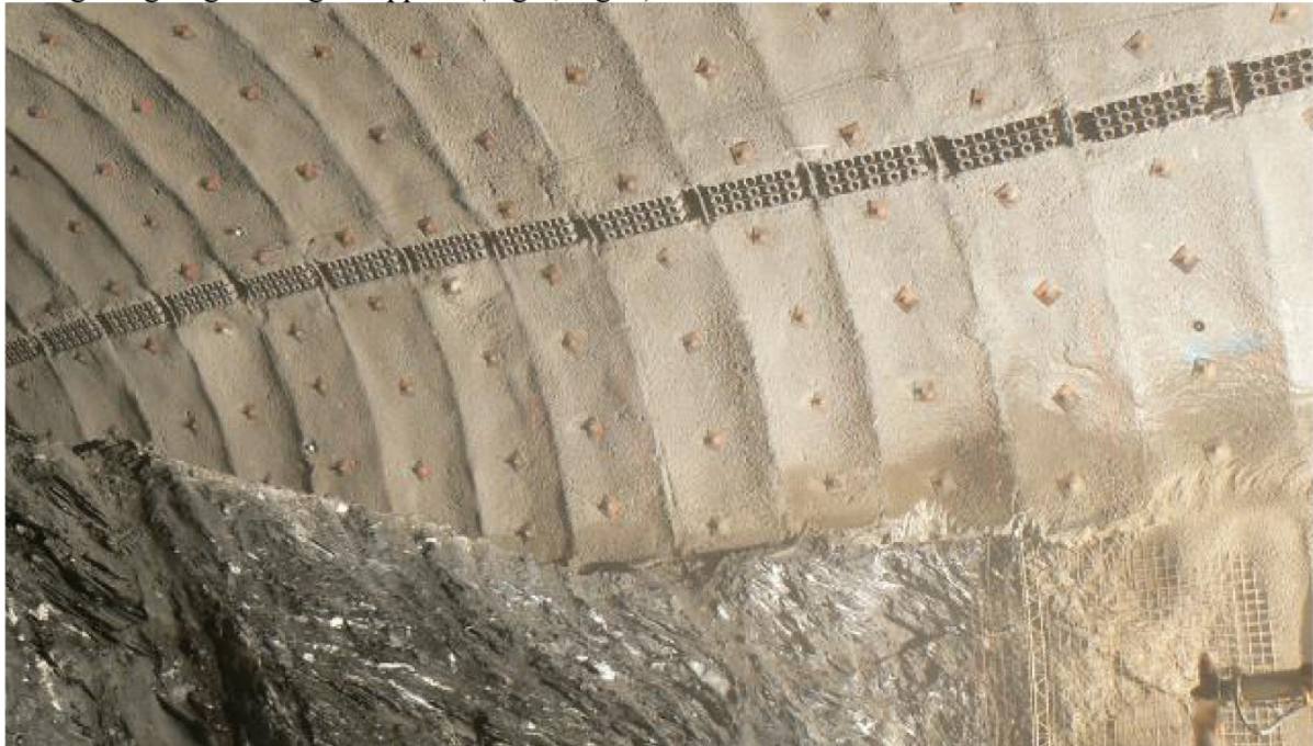
Fig. 1: Grid girder rigid support with compression elements [Bochumer Eisenhütte GmbH & Co. KG]
